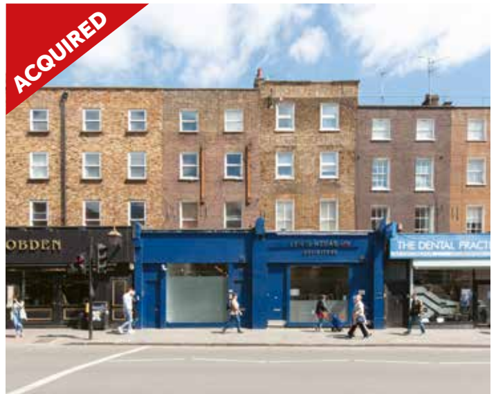
Mixed-Use Investment Camden High Street, Camden, NW1
